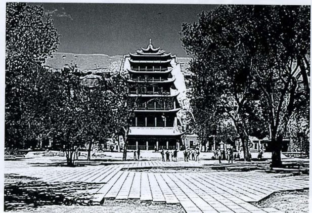
The nine-storey pagoda at Dunhuang housing a massive Buddha statue, with landscaping and paving in progress.
